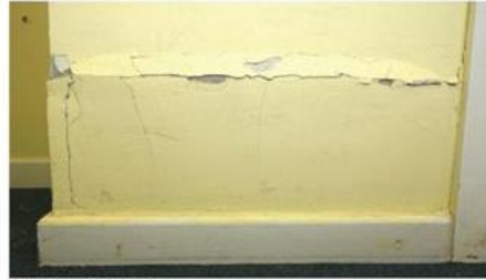
Damage Type 4 Cracking and Buckling of internal partition
